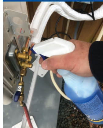
FIGURE 3 Applying a leak-testing solution to newly made flares.
